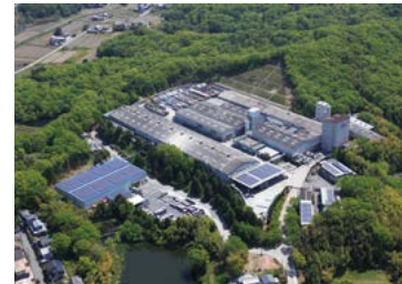
Hyogo Factory mega solar
