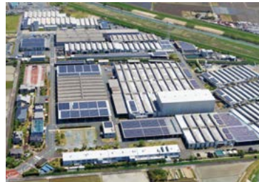
Shizuoka Factory mega solar
