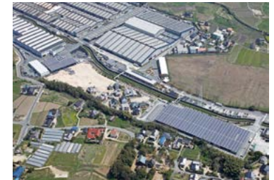
Yamaguchi Factory mega solar
